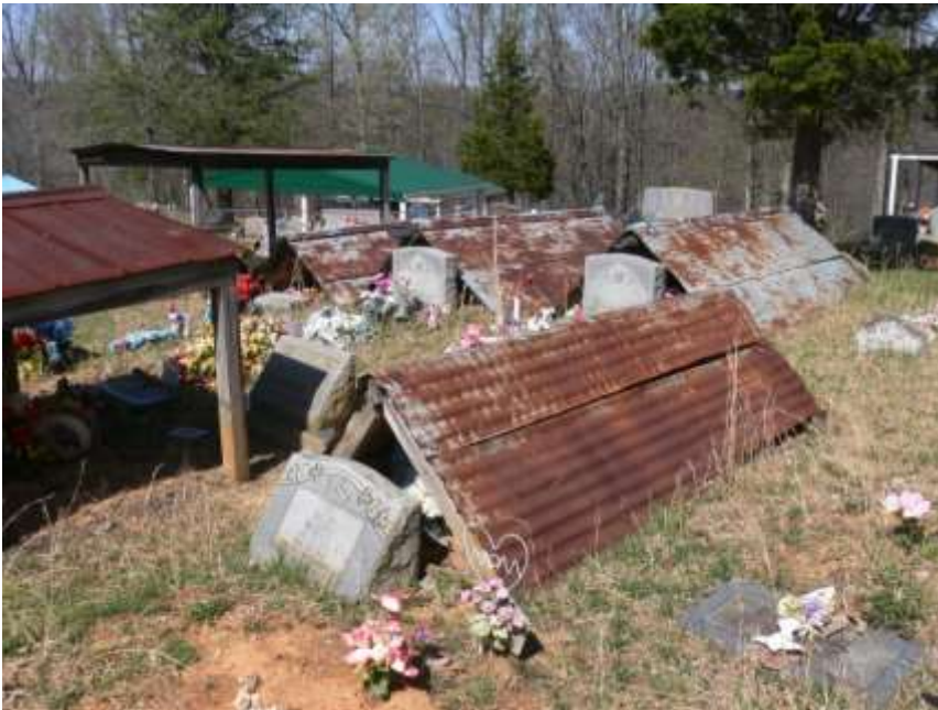
Four of Newsome Ridge Cemetery's five combs of metal roofing.
