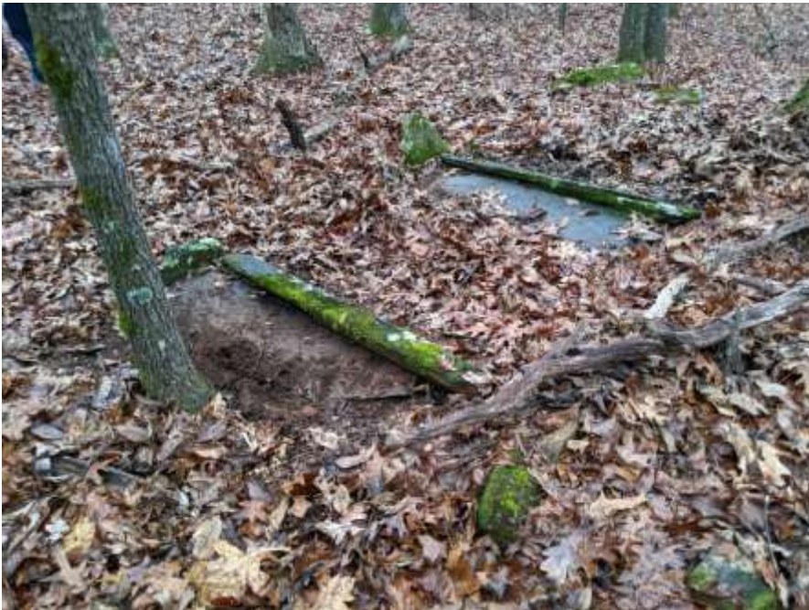
Although partly collapsed, the original gable roof form of the Old Salem combs is evident.
